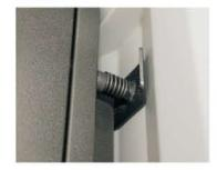
Panel stabilizer feet fall into place along container wall indentation. Secure instadivider panels
