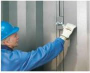
Insert carriage bolts with lock nuts. This secures the insta**divider** panels in place.
