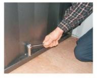
For extra security and strength install lag bolt to the floor.
