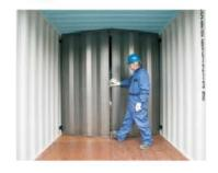
Form a V with the two panels the press into place.
